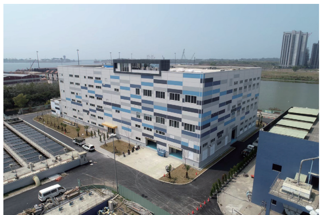
▲ Figure 2-14 Reclaimed water plant in Anping, Tainan
