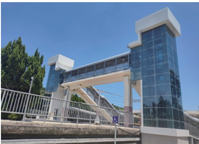
▲ Figure 2-24 Work was completed to elevate the passenger platform at Tsaochiao Station
